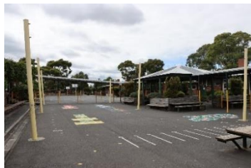
Asphalt – Little house to 5/6 Playground
